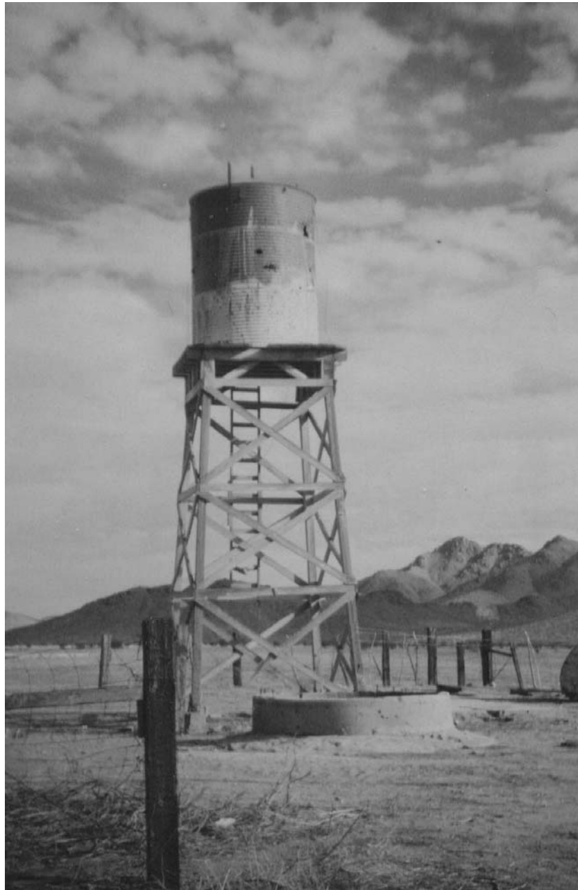
LABPL Water tank – 1963 – Riddled with bullet holes
