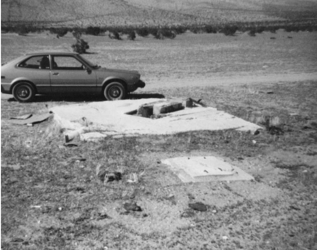
Well in 1981. Note original 1913 engine mount in foreground.
