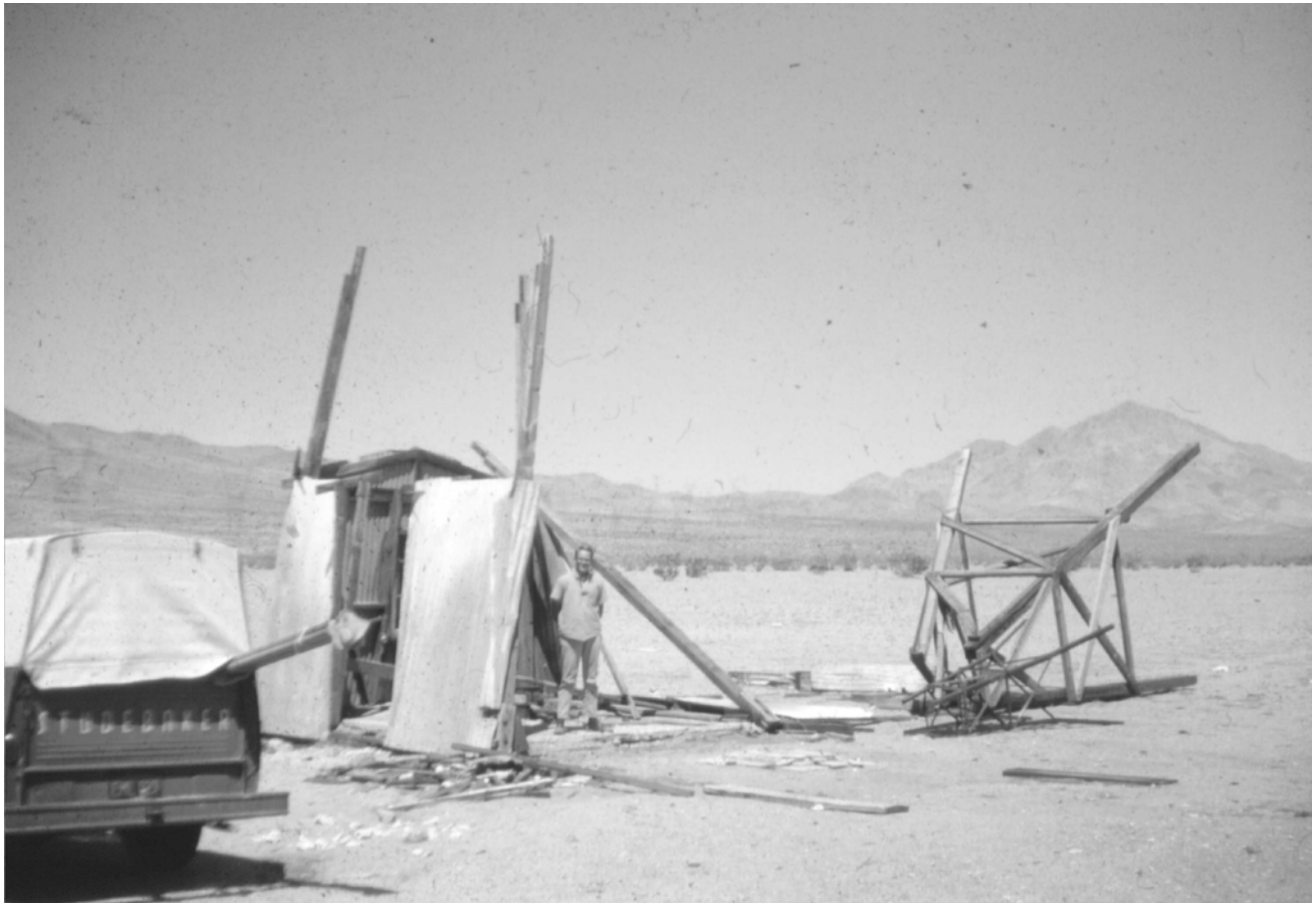
Remains of LABPL Pumphouse - 1963
