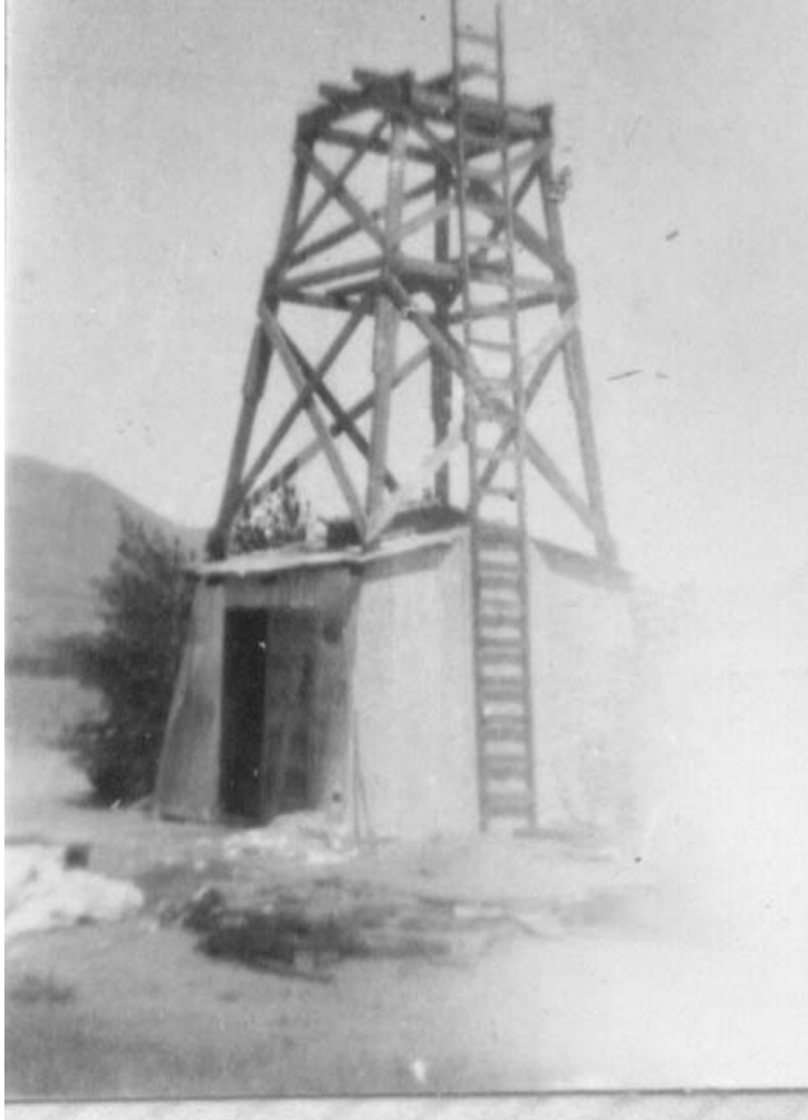
Pumphouse built by LABPL
