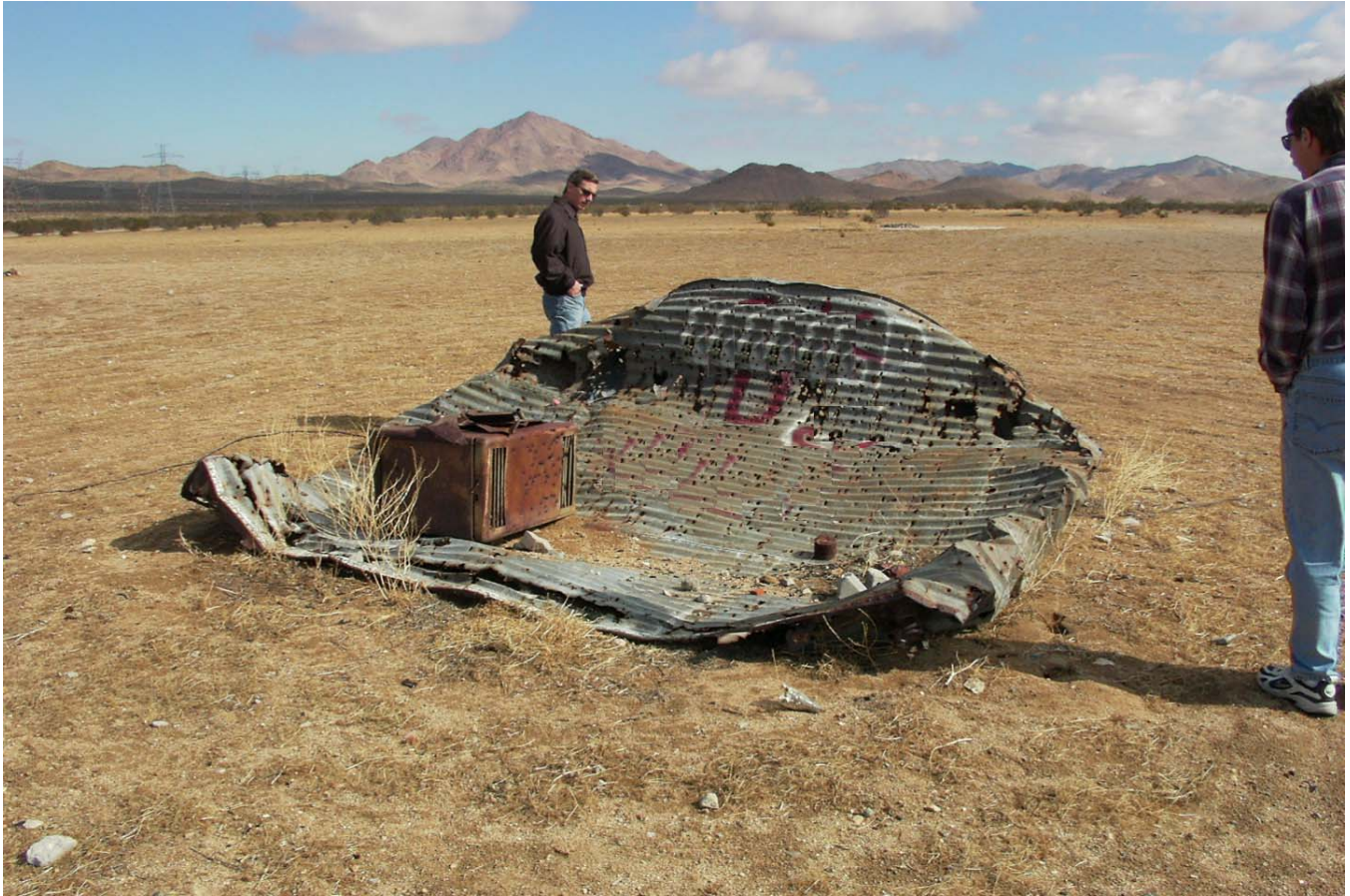
Remains of LABPL water tank - 2003
