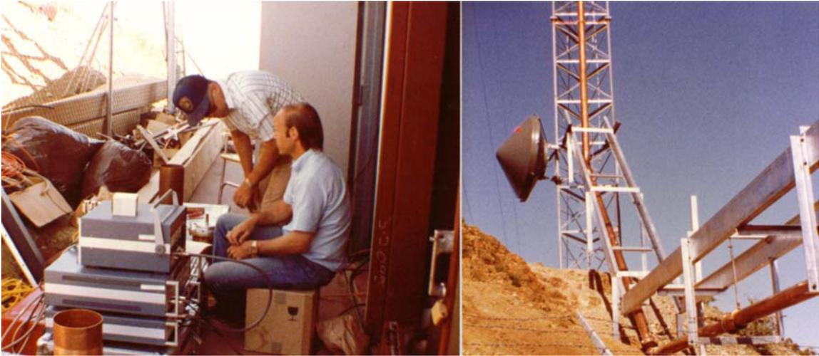
RCA Field Engineer performing proof-of-performance and coax bridge installation.
