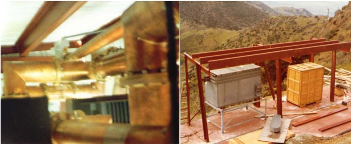
We actually mounted the heat exchanger and set the transmitter on the floor slab and built the building around it.
